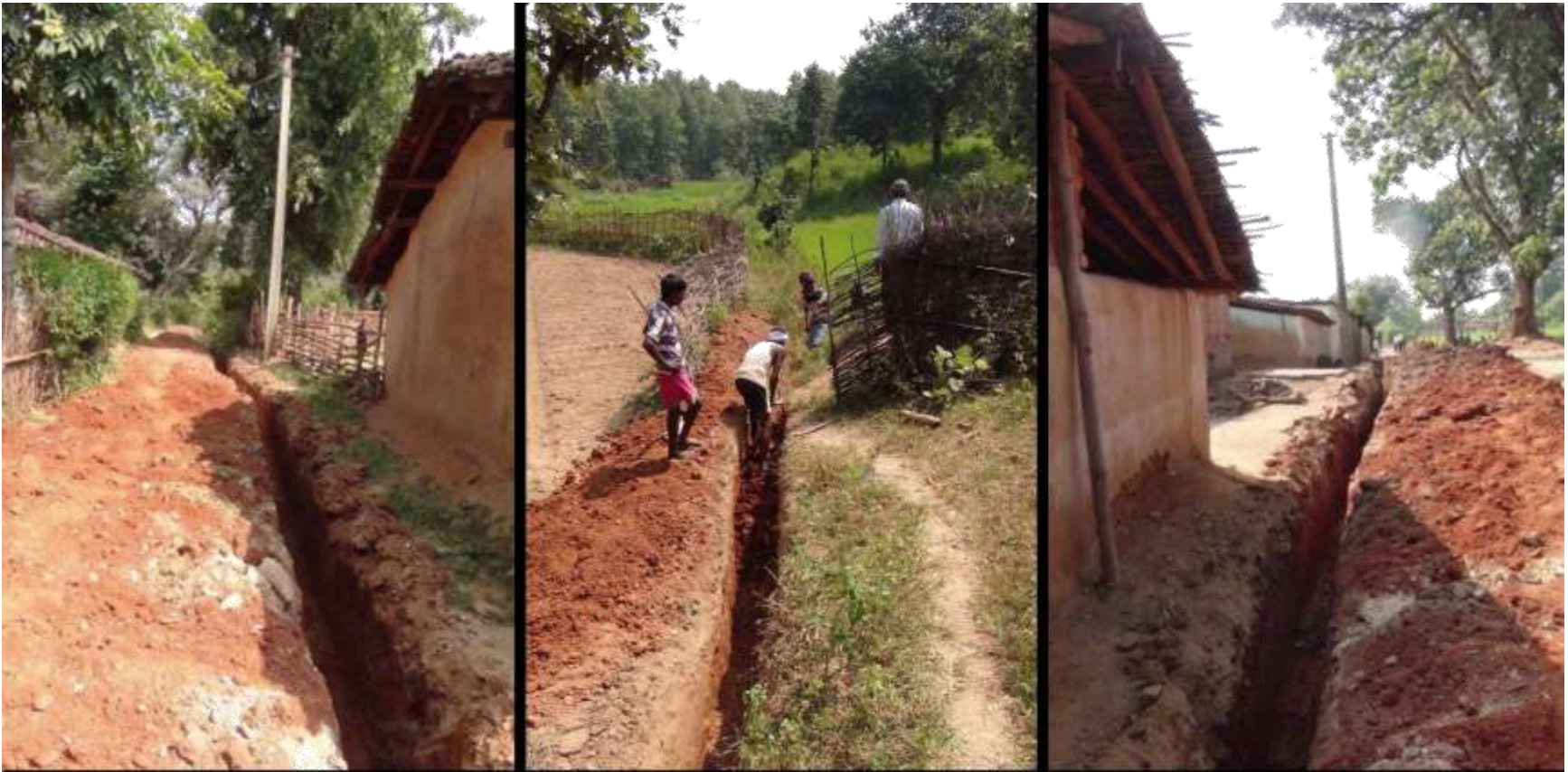
Excavation work for Pipes and Cables trench under progress
