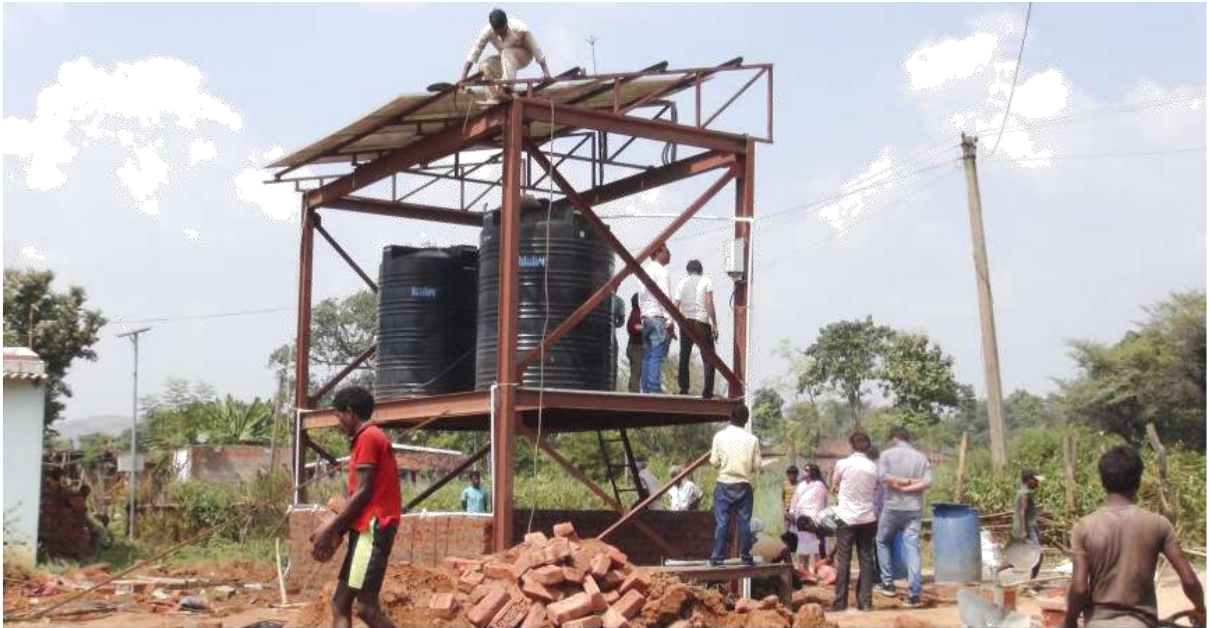
Erection of Solar Panels and construction of water distribution platform
